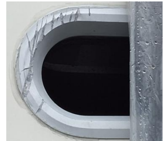
Picture 9 (Left): Inside view of port side bow porthole. Rust stain and corrosion visible on aluminum fasteners. Same condition on starboard side portholes. (not pictured)
