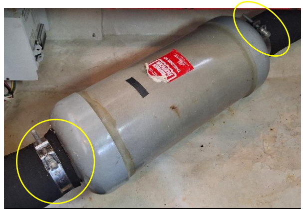
Picture 19: Single hose clamp used at silencer connection.
